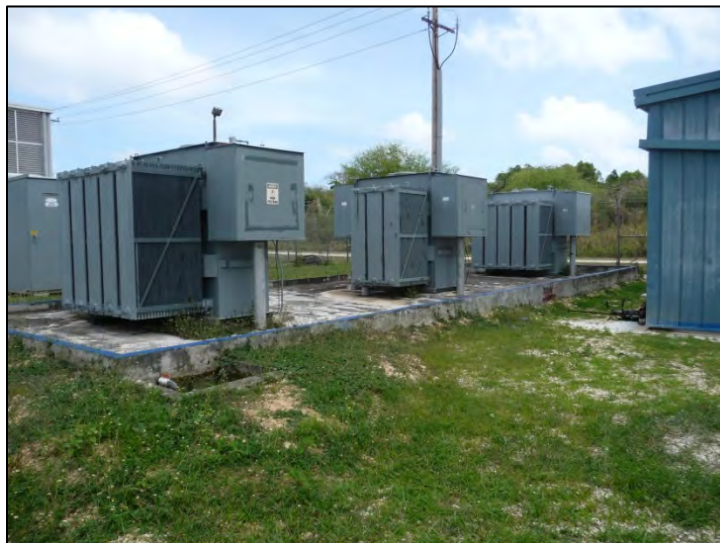
Photo 1.2-3. Power Plant Transformers
