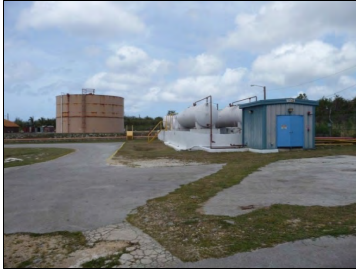
Photo 1.2-2. Fuel Storage Tank (tan) and Lube Oil Tanks (white)
