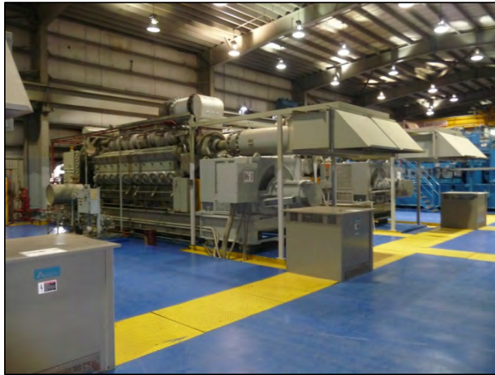
Photo 1.2-1. Tinian Power Plant
